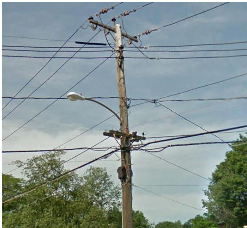
Figure 3: Congested Pole / NEC Clearance Violations - Likely to Require Replacement
