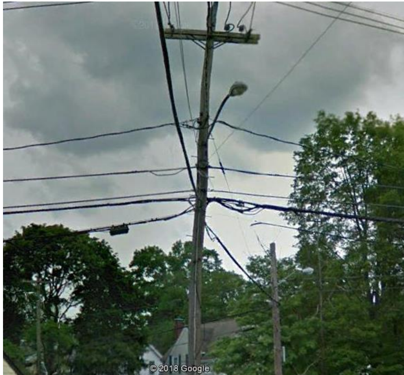
Figure 2: Congested Pole - Make-Ready Will Be Necessary
